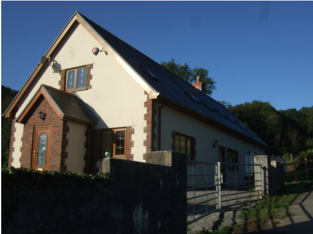
Figure 1: Photograph of the application building – Cildaudy Farm
